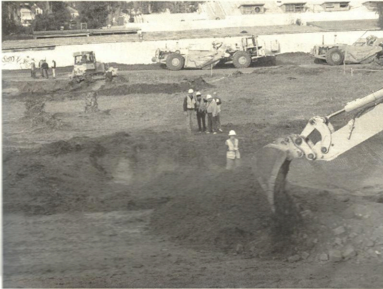
Photo left: Dropping earth and old building bricks in a pile.
