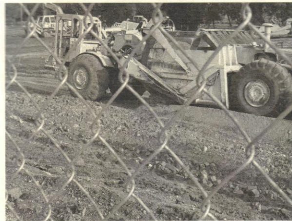
Remains of old Chinatown bricks under the machines
