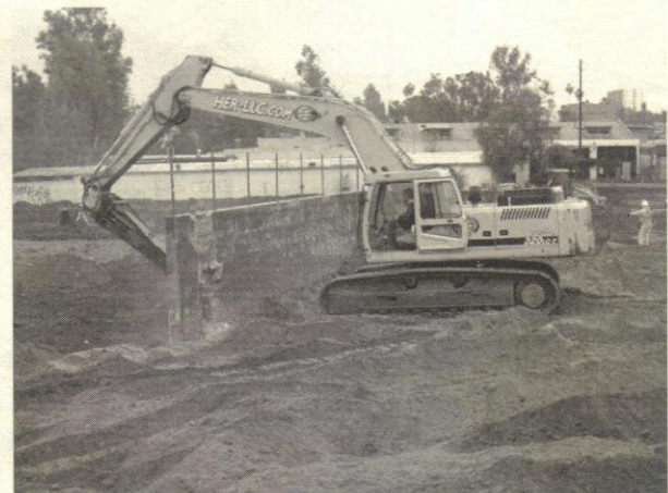
Demolishing a wall
